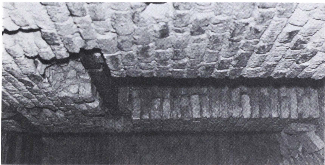
a) Patan, Nārāyaṇa temple, wall core in upper storey
